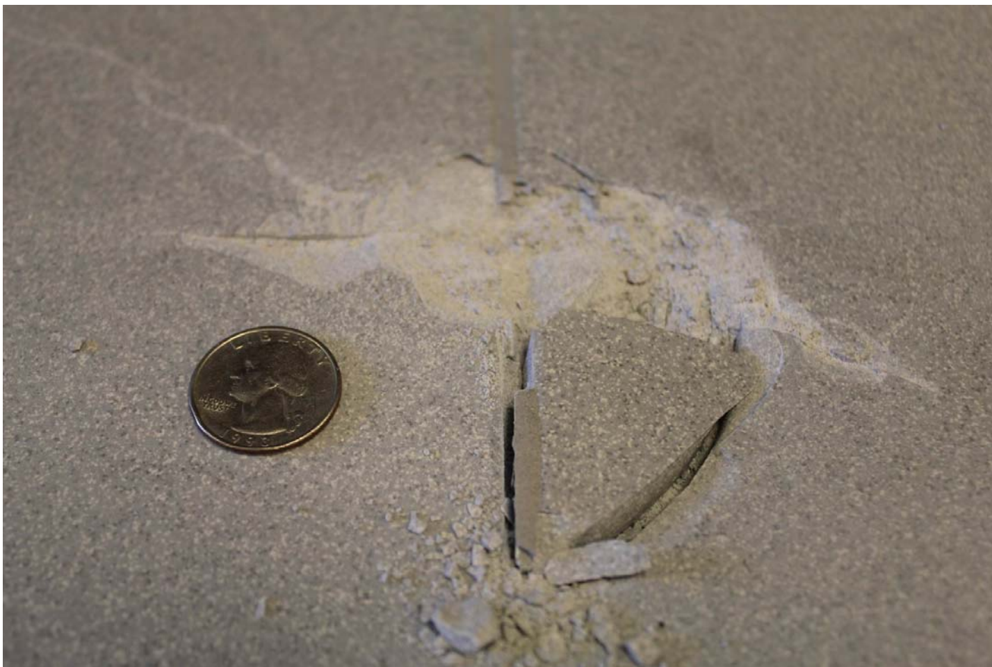
Image 4: Broken tile and spalled grout joint
