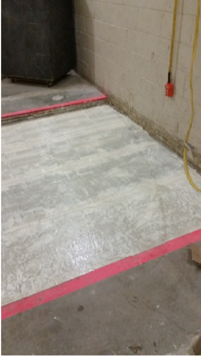
Figure 3 – Adhesive installed on polyethylene sheet over concrete slab
