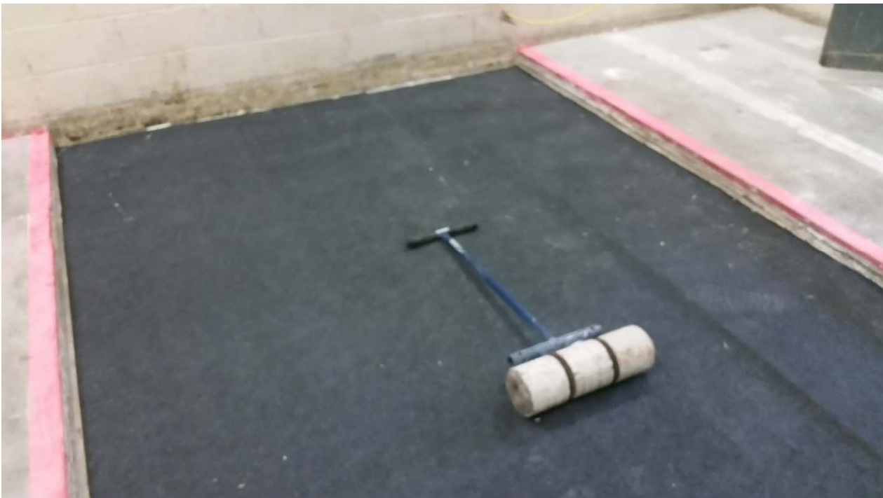
Figure 4 – Underlayment installed, floor roller used in installation
