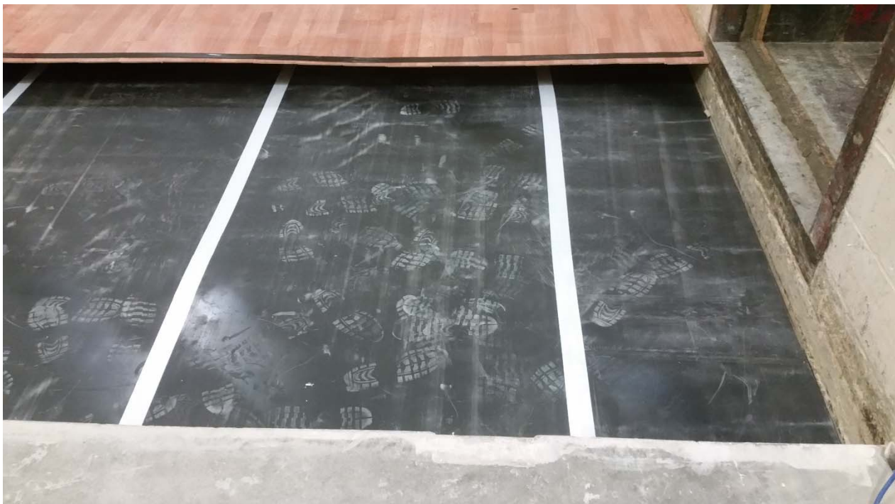
Figure 2 – Underlayment installed over concrete slab
